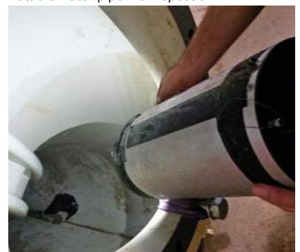
MTA Pipe-Inspector retrieval at Francis turbine
