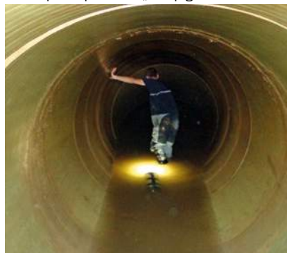
Hydropower pipeline inlet
