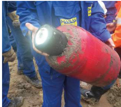
MTA Pipe-Inspector in „taxi pig“
