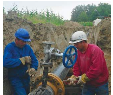
Insertion into gas pipeline
