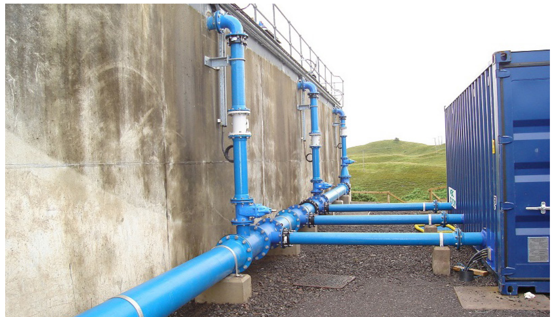
Figure 1. Tullich reservoir with PAX TRS
